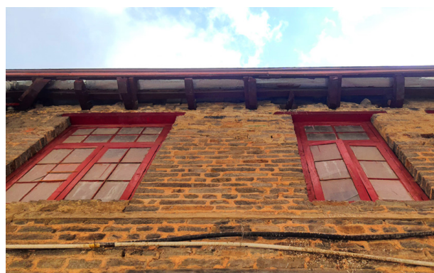
Loose and cracked window glasses pose a threat to the safety.
